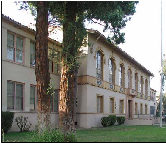
Figure 180. El Sereno Middle School, originally Woodrow Wilson High School (1937). Source: Heumann & Associates and SAIC for LAUSD.
