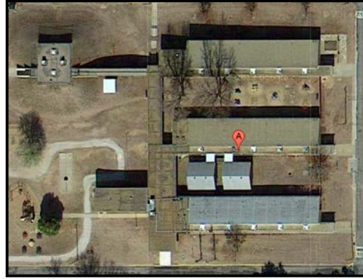
Figure 121. Huston Elementary School, Blackwell, OK. Source: Google Maps, 2013.
