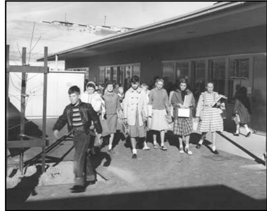
Figure 104. Image for a 1959 article on the “back to back construction” of schools taking place in the San Fernando Valley. Source: LAPL Photos.
