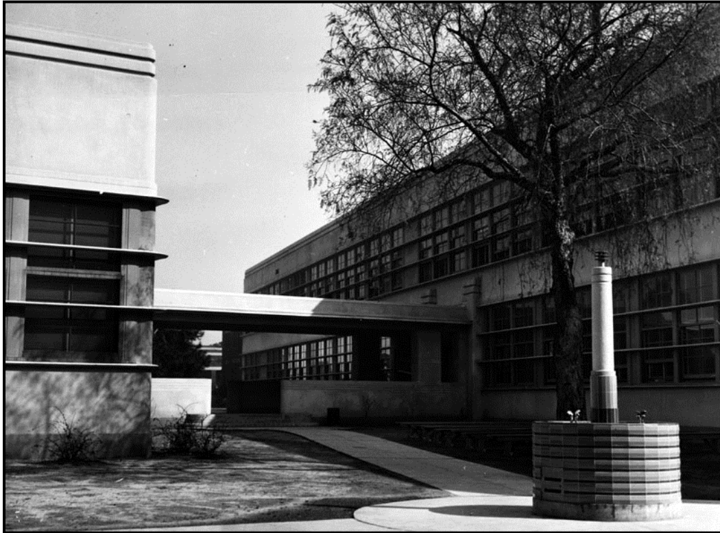
Figure 88. Post-Long Beach earthquake reconstruction at Manual Arts High School, Parkinson & Parkinson, circa 1935. Extant in mid-city Los Angeles, on South Vermont Avenue and West Martin Luther King Jr. Boulevard. Source: LAPL Photo Collection.
