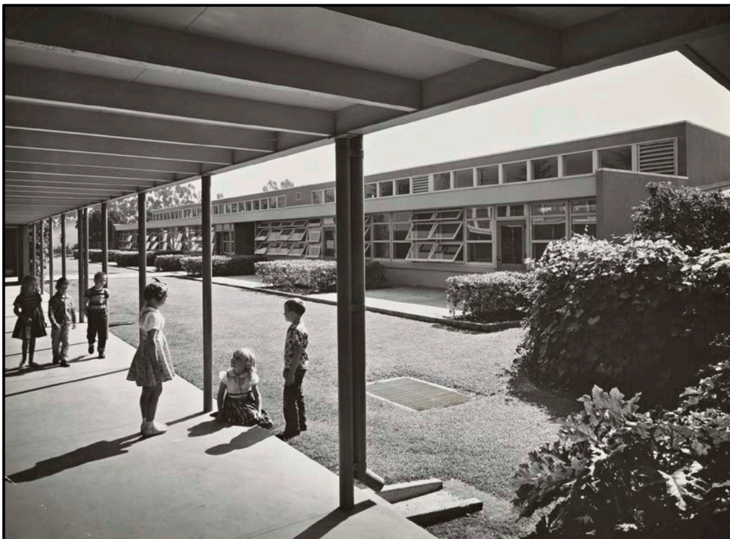
Figure 113. Thomas Jefferson Elementary School, with covered corridors, outdoor courtyard spaces, ample awning casements and clerestories. A sloped shed-roof caps the building for good classroom acoustics. Smith, Powell, & Morgridge, 1954, Anaheim. Source: Getty Research Institute, Shulman Archives.
