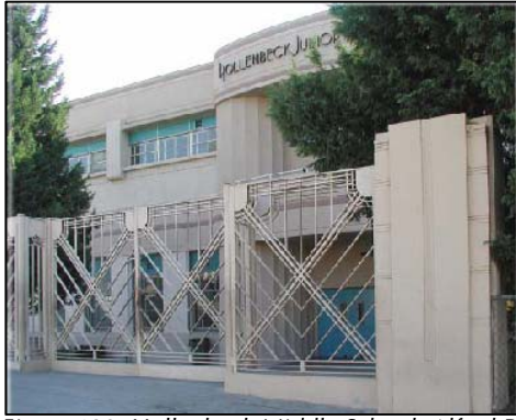
Figure 188. Hollenbeck Middle School, Alfred P. Rosenheim, architect (1936). Source: Heumann & Associates and SAIC for LAUSD.
