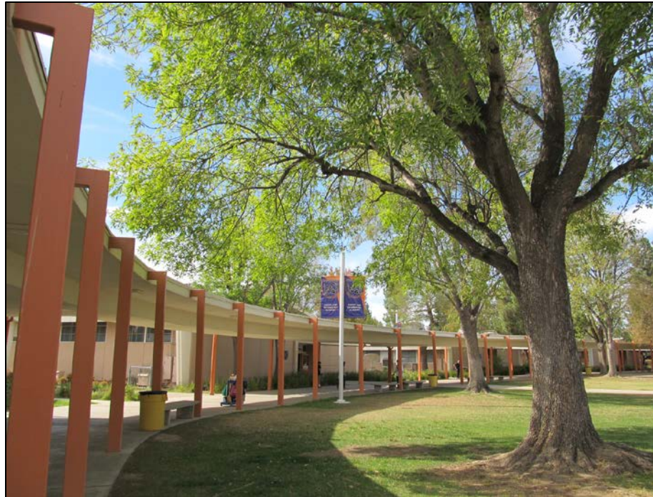
Figure 21. Postwar school: Chatsworth High School (1963), curved outdoor corridor and mature landscaping of student quad and courtyard. Source: Sapphos Environmental, Inc., 2013.
