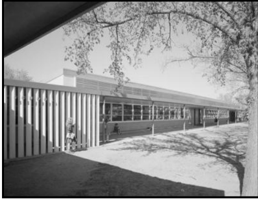
Figure 120. Huston Elementary School, Caudill, Rowlett & Scott, 1949, Blackwell, OK. Source: Getty Research Institute, Shulman Archives.
