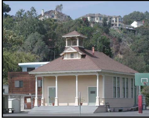
Figure 170. Old Canyon School (1894). Source: Heumann & Associates/SAIC for LAUSD.
