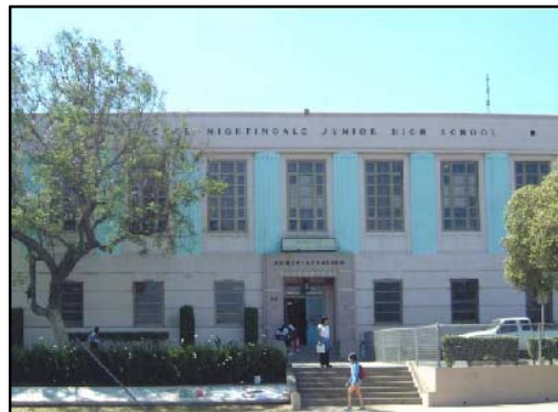
Figure 185. PWA Moderne with Art Deco influence: Florence Nightingale Middle School, John C. Austin & Frederick M. Ashley, architects (1937-1939). Source: Heumann & Associates and SAIC for LAUSD.
