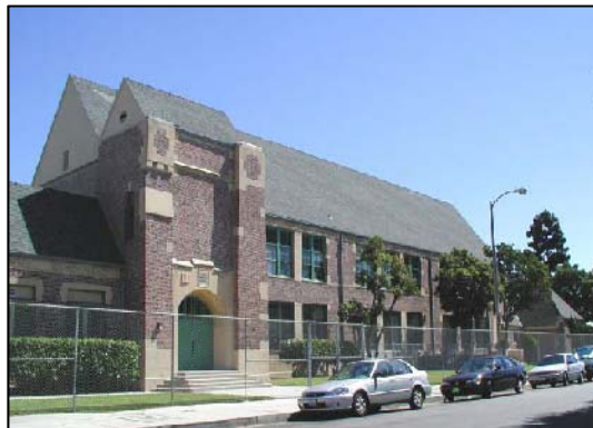
Figure 202. Gulf Avenue Elementary School, Henry Harwood Hewitt & Norman Miller (1926). Source: Heumann & Associates and SAIC for LAUSD.
