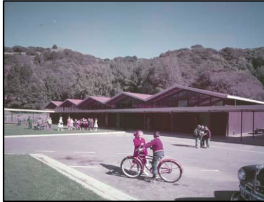
Figure 106. John Lyon Reid, Manor Elementary School, Fairfax, California, 1958. Source: J. Paul Getty Trust, Getty Research Institute, Shulman Archives.
