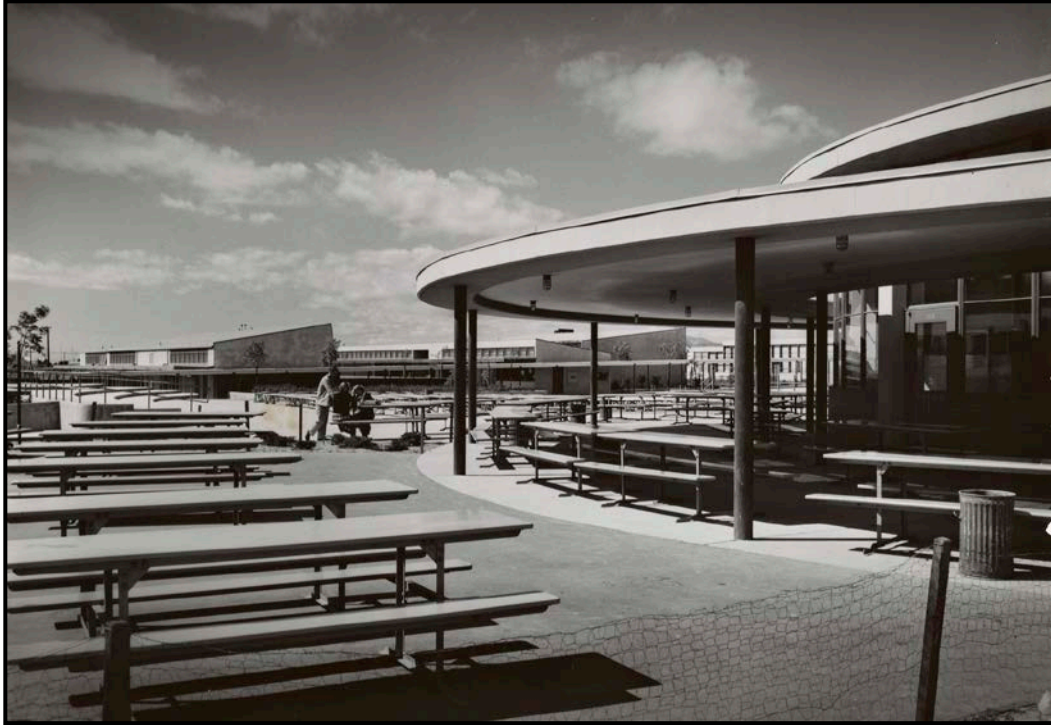
Figure 134. Orville Wright Middle School (originally Westchester High School), Spaulding & Rex, 1948-1952. Source: Getty Research Institute, Julius Shulman Archive.
